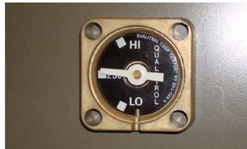
Figure 5. Liquid level gauge
